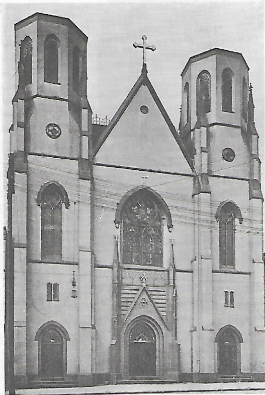
Exterior of Saint Lawrence Church Walnut Street at Fifth
